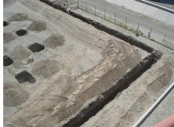
Cut-Off Trenches / Pre-Excavated Pillars
