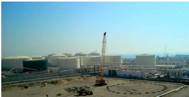
Ring trench DC at Tank TK-10
